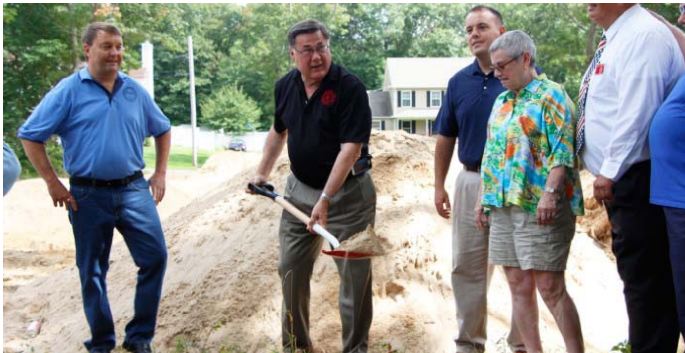
Supervisor Ed Romaine breaks ground where the two homes are being built for returning veterans. Photo by Giselle Barkley
